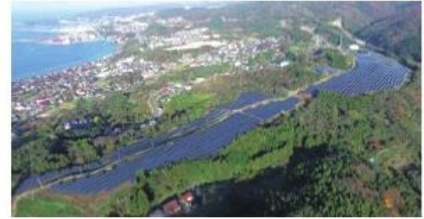
The 12MW solar power plant in Hamada in Shimane Prefecture Japan
